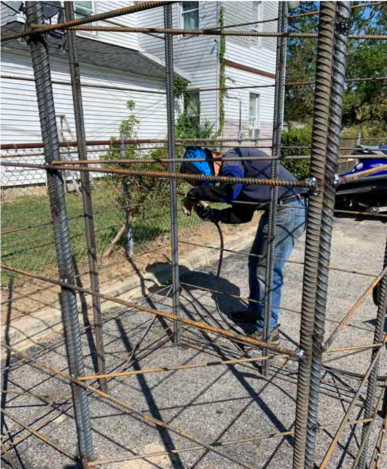
W2YW Welding the rebar cage for the HDX 572 tower
